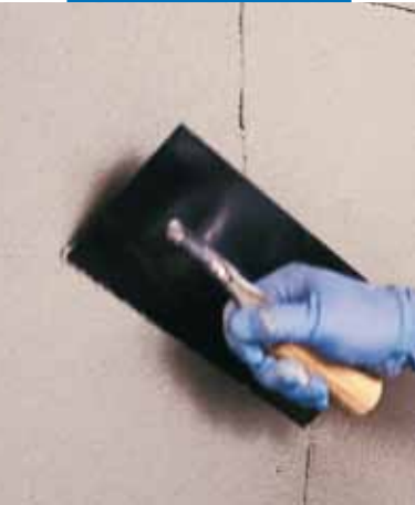
Applying Planitop 560 with a metal trowel
