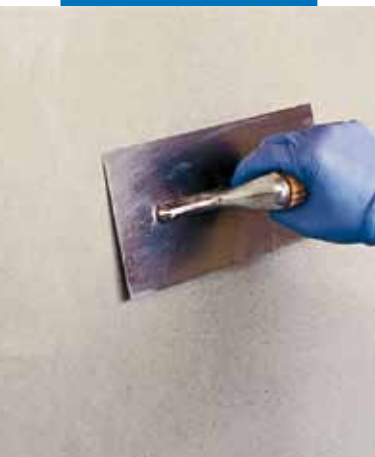
Smoothing Planitop 560 surface with a metal trowel
