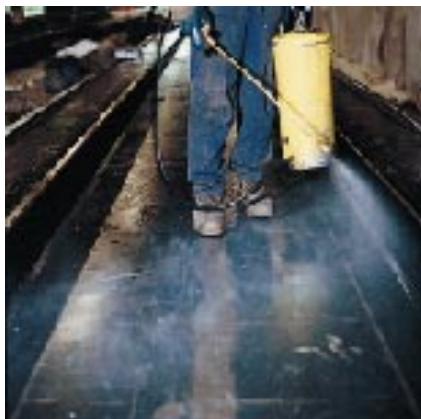
Spray application of DMA 2000 FORM-RELEASE AGENT
