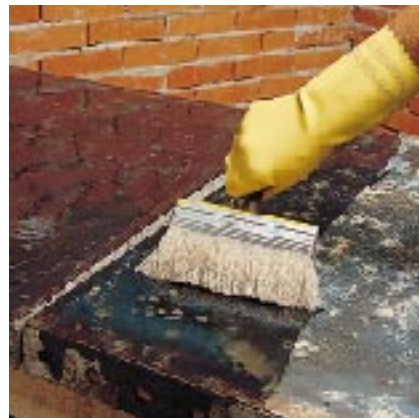
Applying DMA 2000 FORM-RELEASE AGENT with brush
