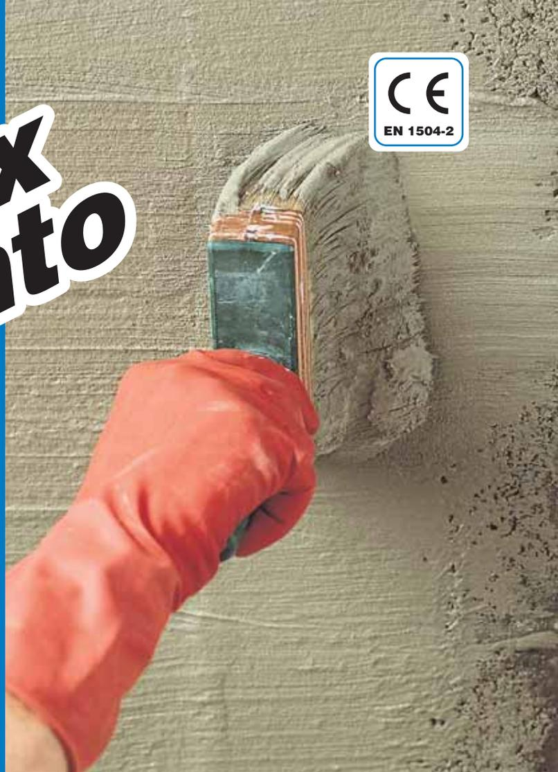
**Osmotic cementitious mortar suitable for contact with drinking water, for waterproofing masonry and concrete structures**
