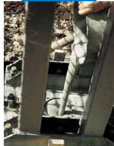
Anchoring of metallic carpentry with Mapefill
