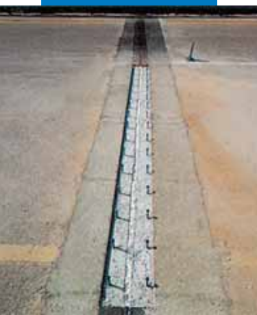
Repairing rigid joints of a highway bridge with Mapecfill
