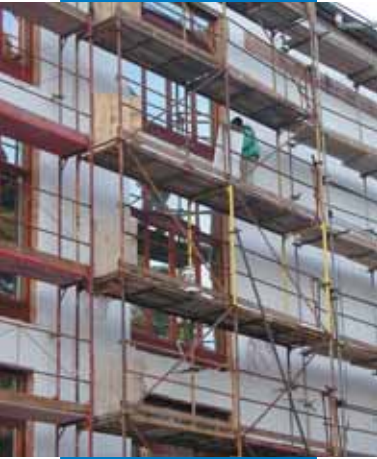
Bonding the insulating blocks to the façade with Mapetherm AR1
