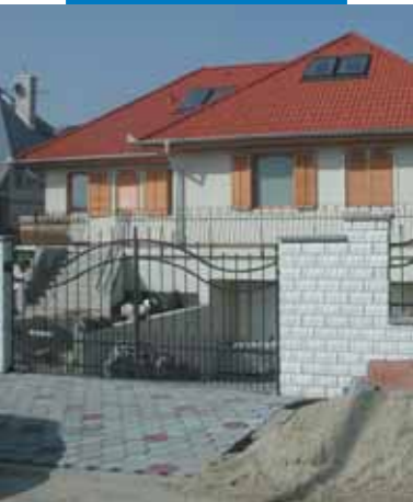
Private villa with foamed heating insulation - Hungary
