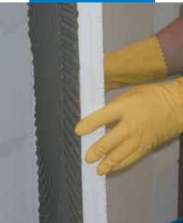
Installing the insulating panels
