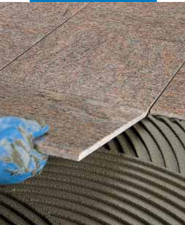
Installation of pre-glossed marble on floors
