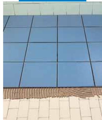
Tile on tile with Keraflex grey
