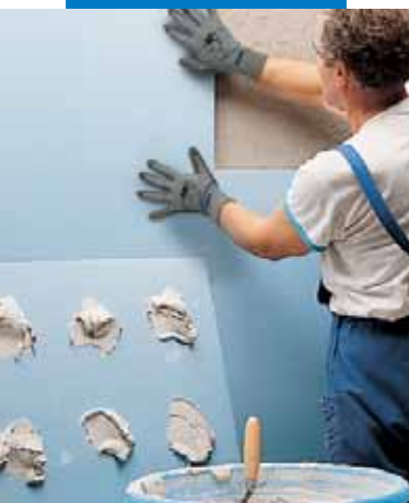
Laying polystyrene foam slabs with Keraflex white
