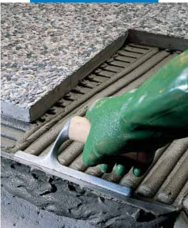
External installation of relief terrazzo "graniglie" tiles
