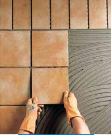
External installation of klinker tiles
