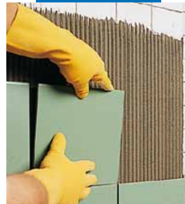
Laying over old tiles
