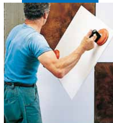
Laying KERAION on a wall
