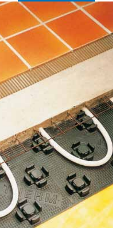
Laying over an underfloor heating installation
