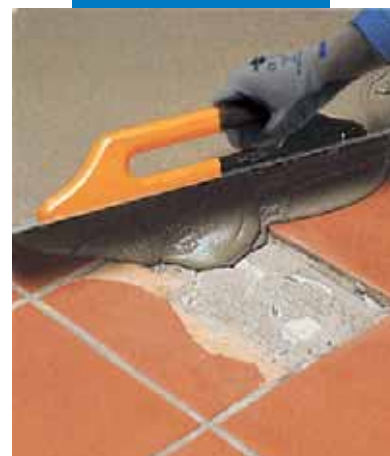
Filling holes with Nivorapid
