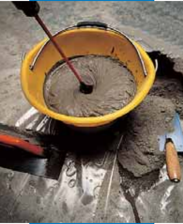
Nivorapid mixed with mechanical mixer
