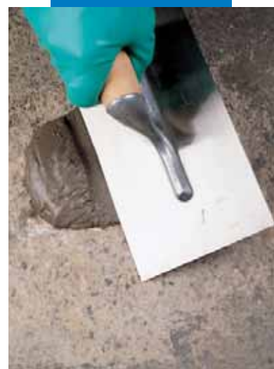
Repairing horizontal arrises with Nivorapid
