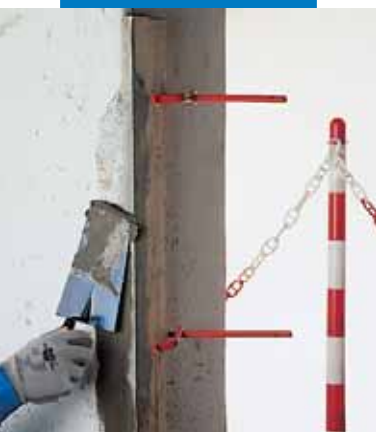
Repairing vertical arrise with Nivorapid
