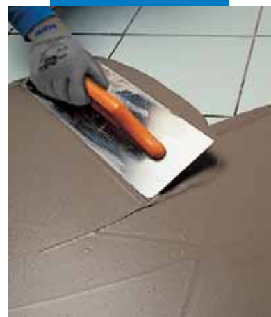
Levelling of existing floor with Nivorapid
