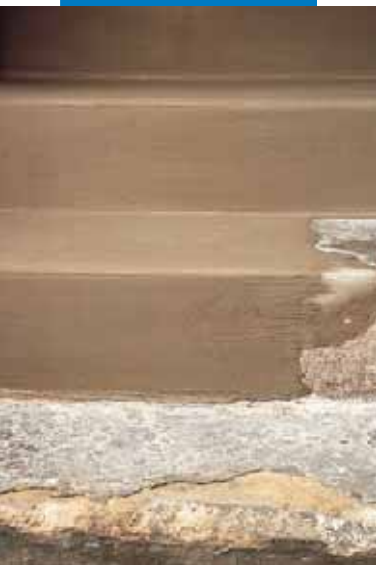
Steps before and after being treated with Nivorapid
