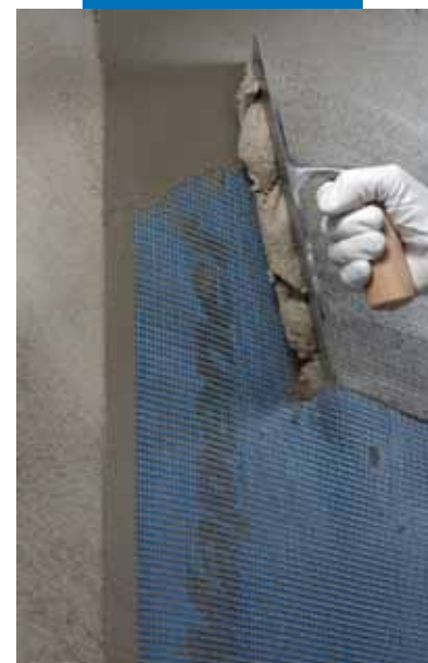
Application of the second layer of Planitop 200 on a substrate made from different materials with Mapenet 150 embedded between the layers
