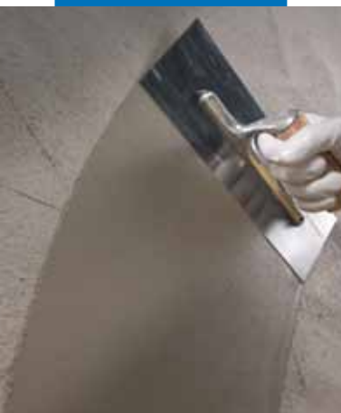
Applying Planitop 200 on concrete
