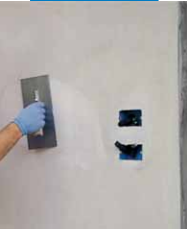
Applying Planitop 520 with a metal trowel
