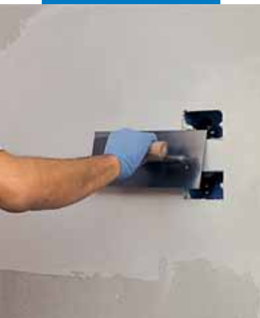
Applying Planitop 520 with a metal trowel
