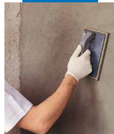
Finishing the Planitop 540 surface with a sponge float
